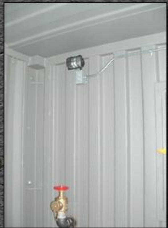
INTERNAL STAIRS WITH LIGHTING AND STANDPIPE CONNECTIONS
