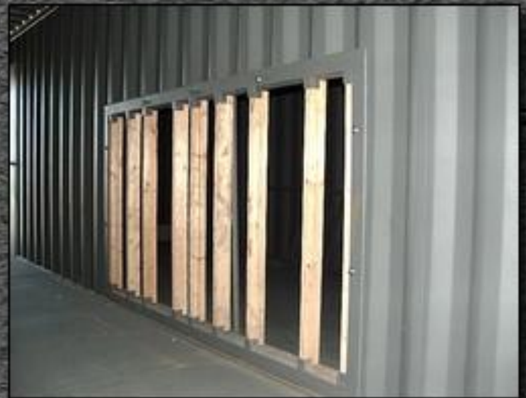
WALL BREACH PROPS
